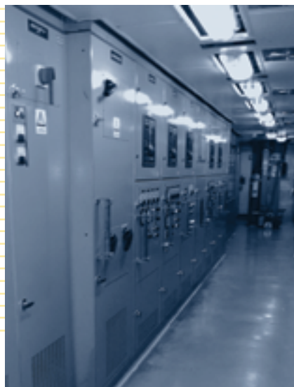
SCR/MCC room on offshore rig
