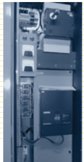
SCR drive on offshore rig
