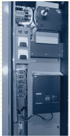
SCR drive on offshore rig
