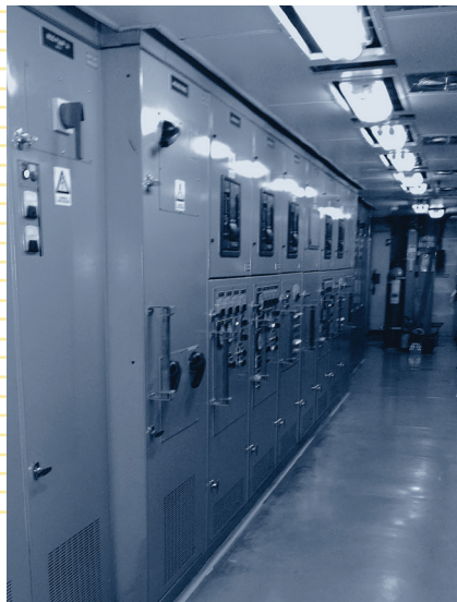
SCR/MCC room on offshore rig
