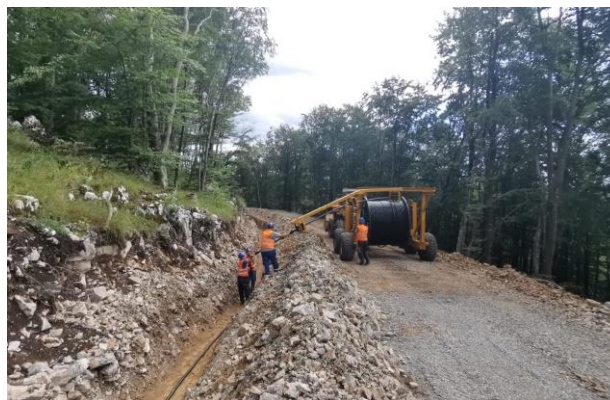
Machine for automated cable laying
