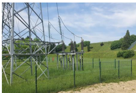
SS Machine room HPP Varaždin
