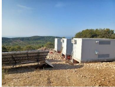
Vis solar power plant
